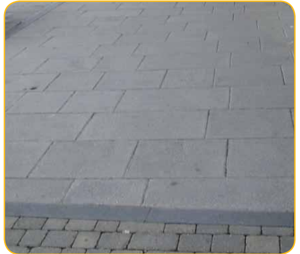
Marshall's Natural Saxon 450 x 600mm rectangular slabs
