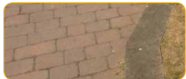
Marshalls Tegula block paving in various colours (eg Market Square)
