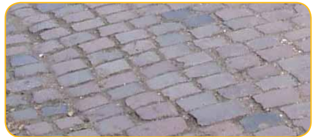
Granite Setts (eg Mill Lane)
