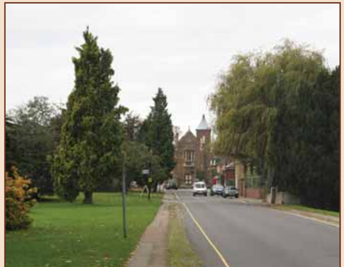
Trees enclose the view west along Park Street
