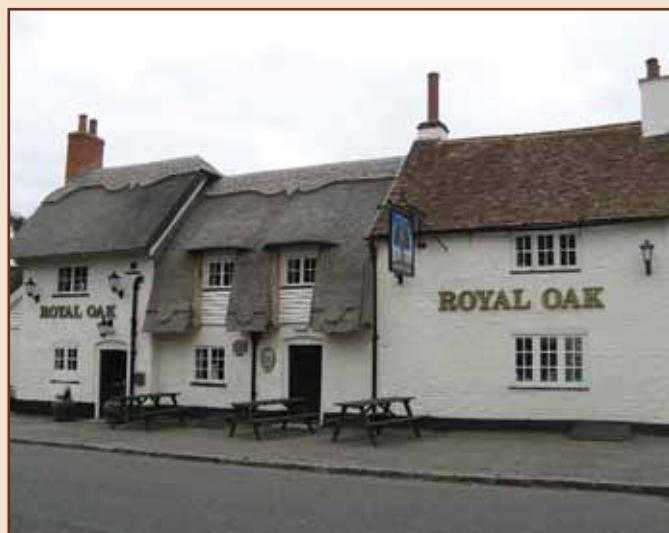
Royal Oak public house, George Street – thatch, old tile and lime plaster
