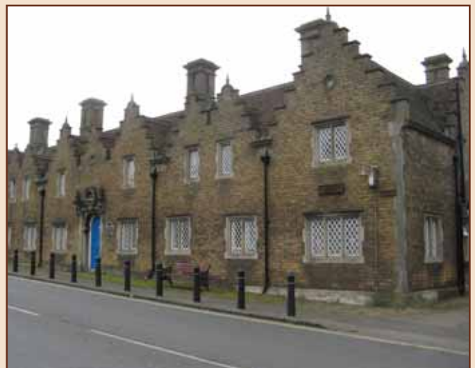
Staunton House, Bedford Street
