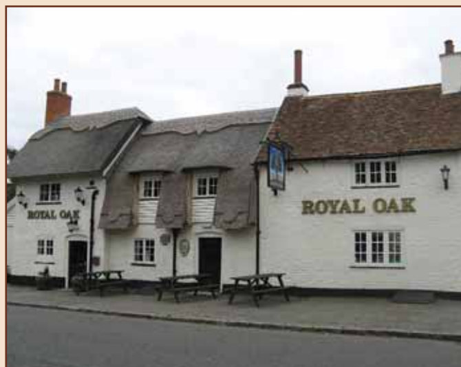
Royal Oak public house, George Street – thatch, old tile and lime plaster
