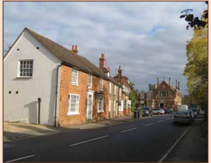
View east along Leighton Street to the Town Hall
