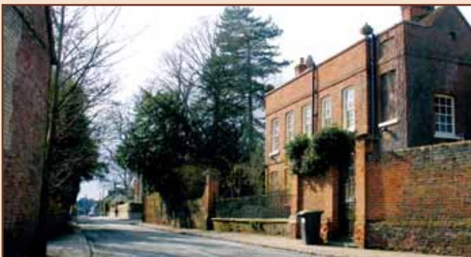
Clophill House: Formal, urbane and striking
