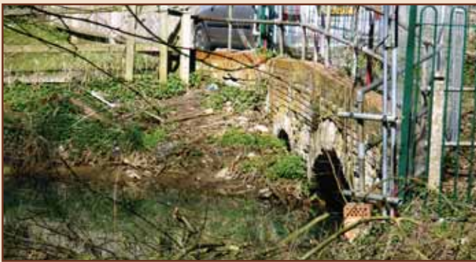
The arches of the old ironstone road bridge
