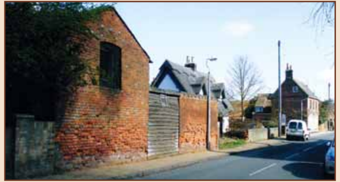
North side of the High Street weathered brick walls
