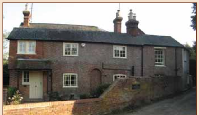
Enclosure created unusually by an oblique brick wall boundary
