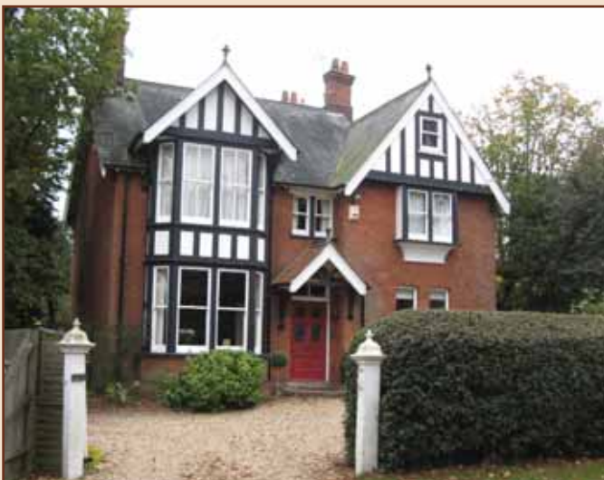
A typical interesting and well-detailed late Victorian house
