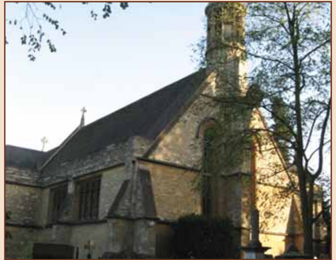
The Church of St Michael (Grade II* listed building)
