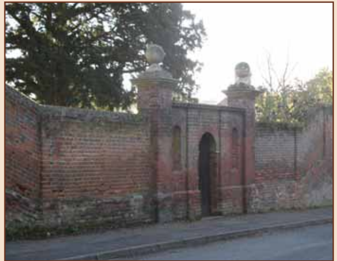
Garden walls to Aspley House
